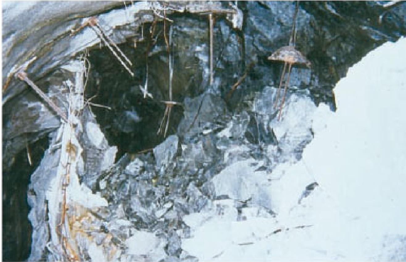
**Figure 3—Rockburst damage showing protruding and failed support elements (photograph W.D. Ortlepp)**
